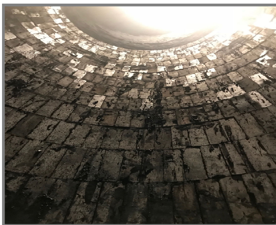
DuraLast NB SiC - Upper or Lower Stack
