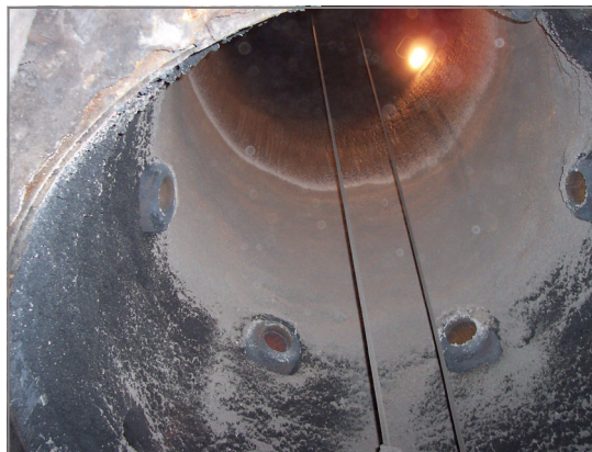
DuraMeltz® Melt Zone shotcreted with Allied Mineral Product Monolithic
