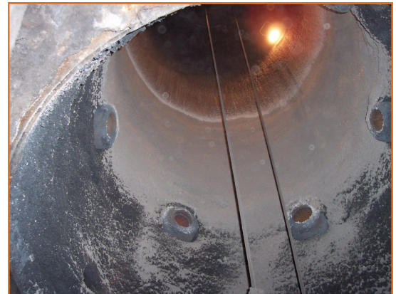
DuraMeltz® Melt Zone shotcreted with Allied Mineral Product Monolithic
