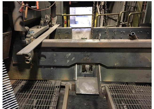
External Air Cooling
